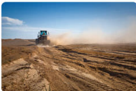
Earth-moving equipment prepares a site for construction. The soil is pushed aside and the land is left bare. Some of the soil blows away even as the machine moves it.
